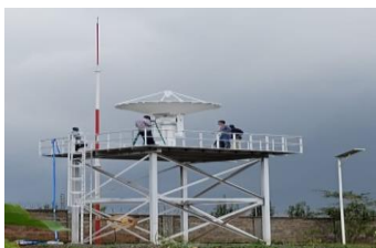
RARS station installed on the roof of AGRHYMET's building (Niamey- Niger)
