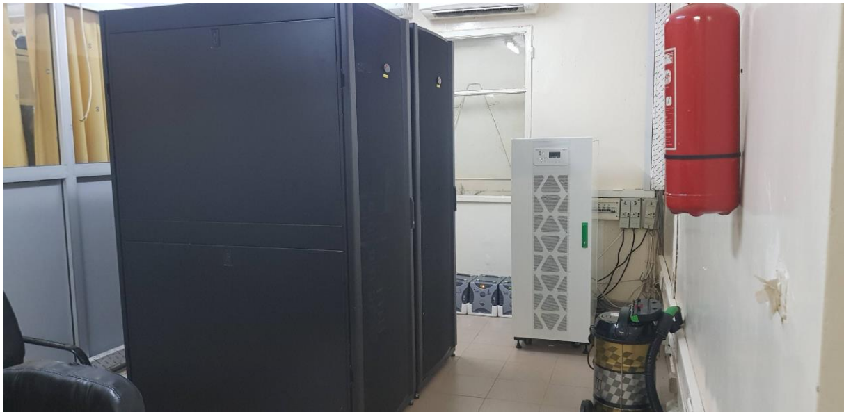
Figure 1: High Performance Computing System installed at ACMAD with 344 cores and 600 Terabytes of storage capacity.
